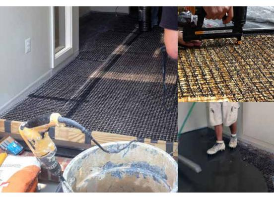
Traditionally tile struggles to offer good impact noise resistance in flooring applications. Since impact noise travels through connections, tile tends to perform poorly compared to carpet or other hard surfaces. Dependable offers a unique solution to this problem: QQ Step Soft™.
