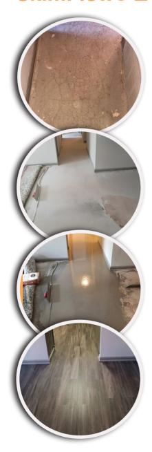
After a multi-family project experienced product failure and loss of time, the job needed an effective solution to reverse the damage done in a timely manner. Johnson's Commercial Flooring turned to FloorPrep.com Primer A to double prime the gypsum concrete sub-straight and underlayment SkimFlow® LCB, with its suitability for finished flooring, such as LVP.
